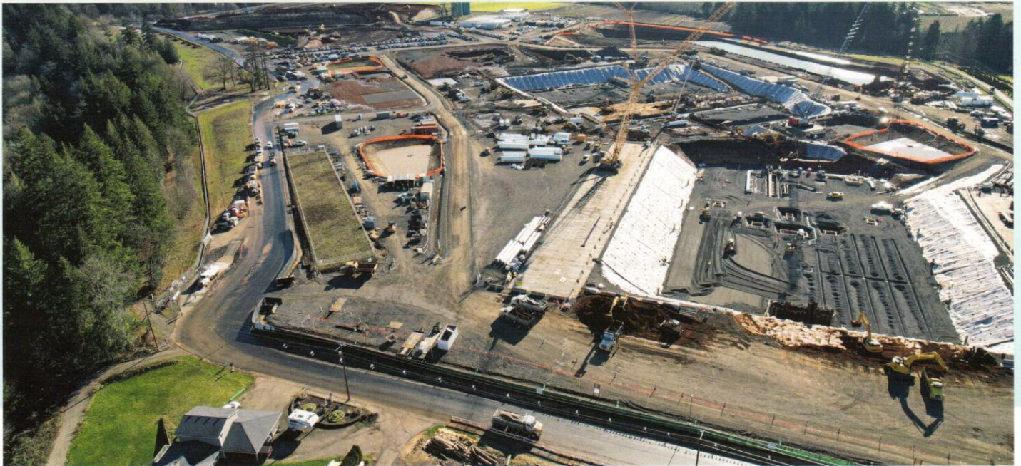
Filtration facility construction progress in early 2025
